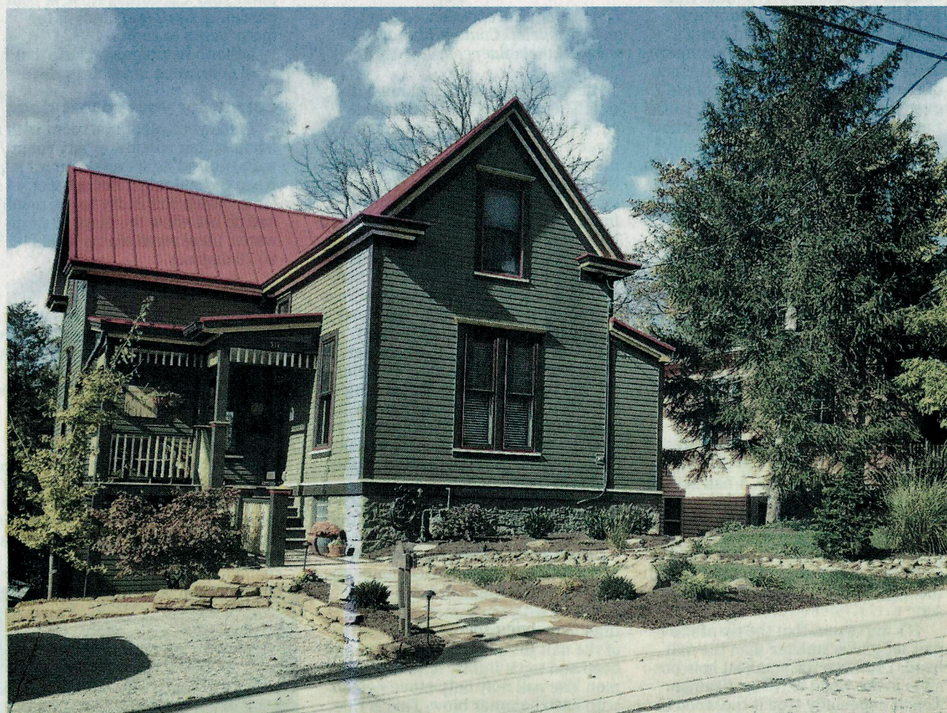
The Nietches agreed on the dark green fiber cement siding, but the red metal roof and trim in various shades of yellow were Kim’s doing. THE ENQUIRER/BRENT COLEMAN
